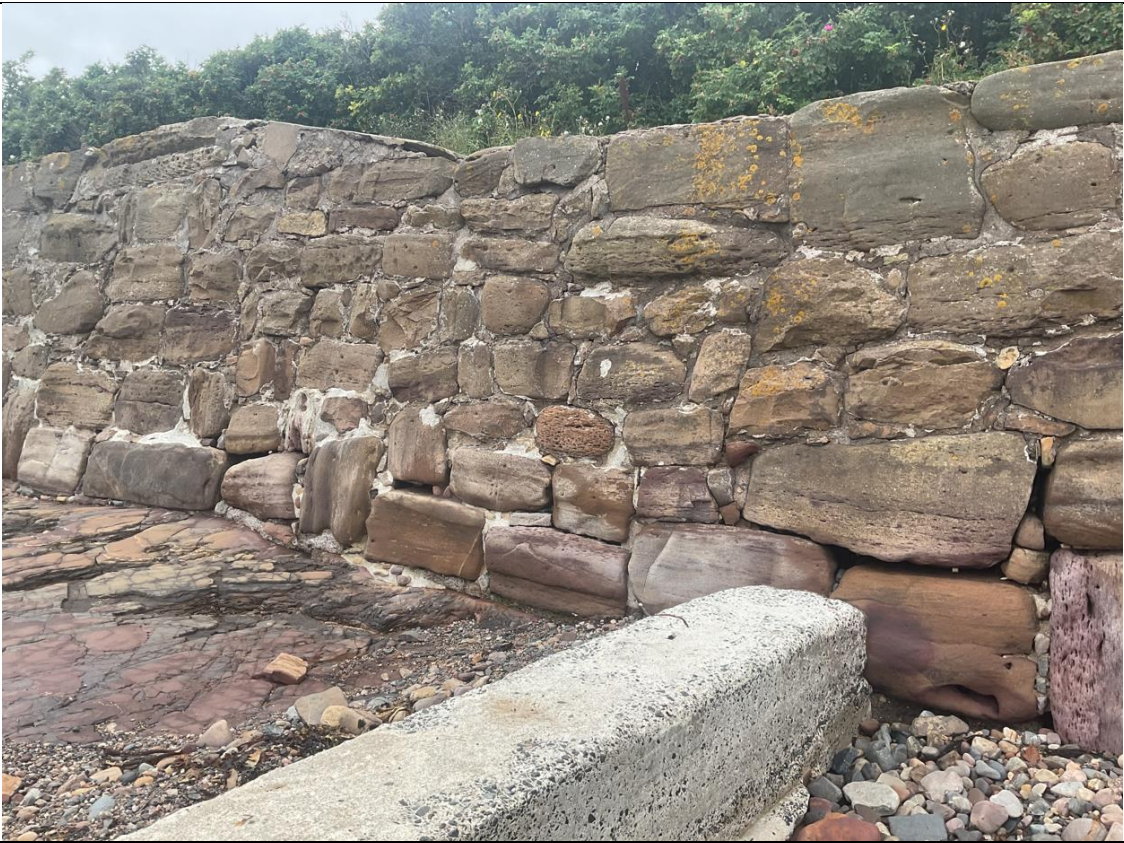
Figure 32- General wall condition approximately between ch396-ch458.
