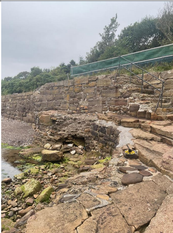
Figure 33- General wall condition at ch458.
