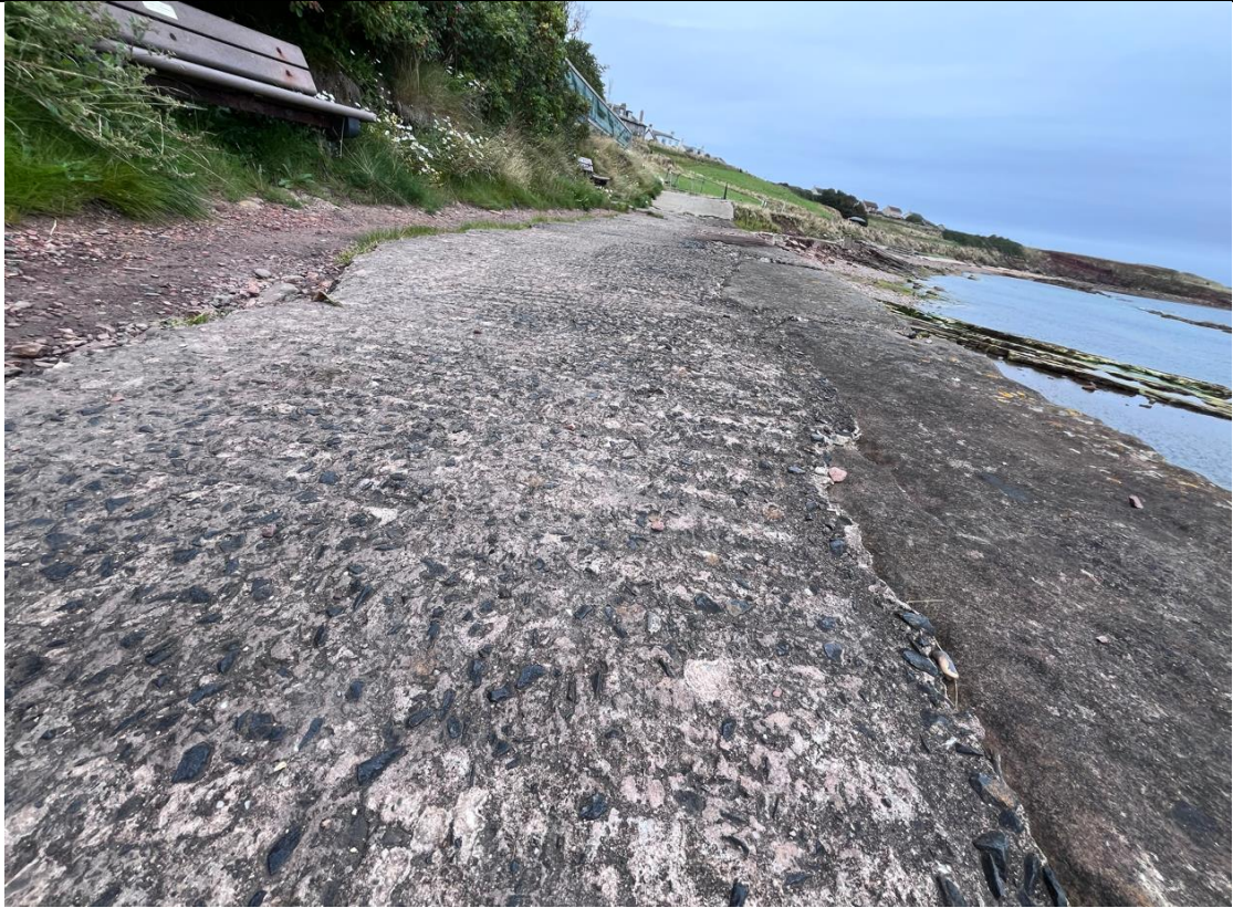
Figure 51- Path surface between ch384-ch414.
