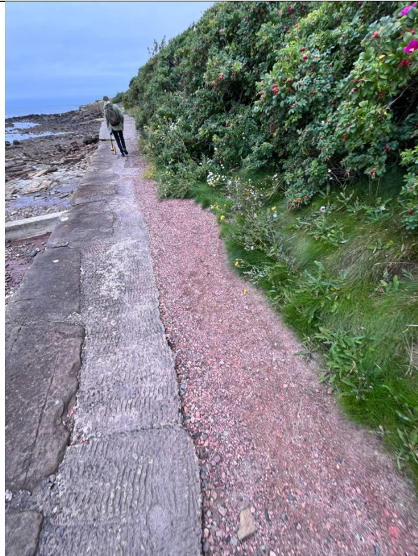
Figure 52- Path surface between ch384-ch414.
