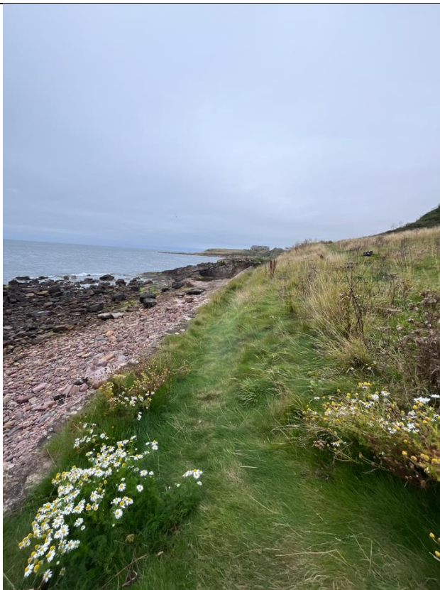
Figure 34- Between ch000-ch65 there is no path/surface cover.
