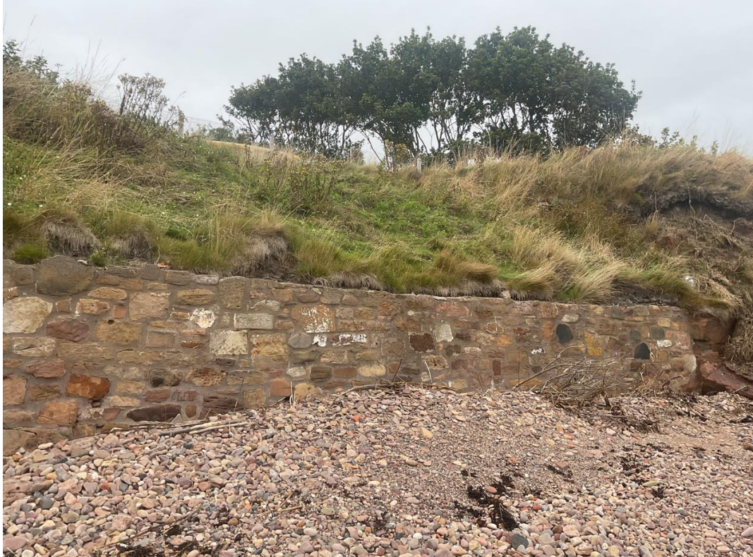
Figure 17- Between ch149-170 a newer section of wall has been constructed.
