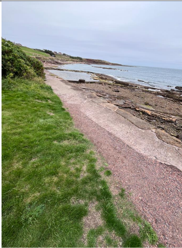
Figure 47- Subgrade material coverage, between ch341-ch349.
