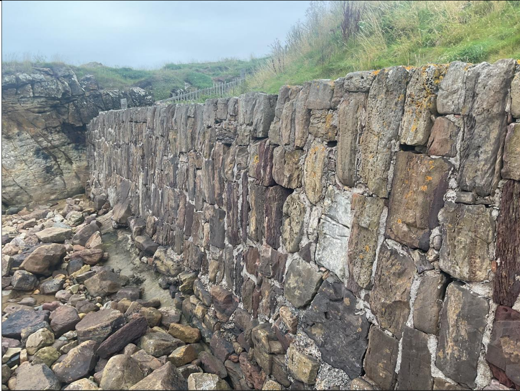
Figure 1- General condition of the wall between ch000-ch23.5.
