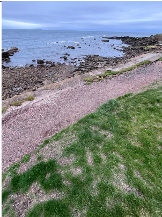
Figure 46- Subgrade material coverage, between ch295-ch341.
