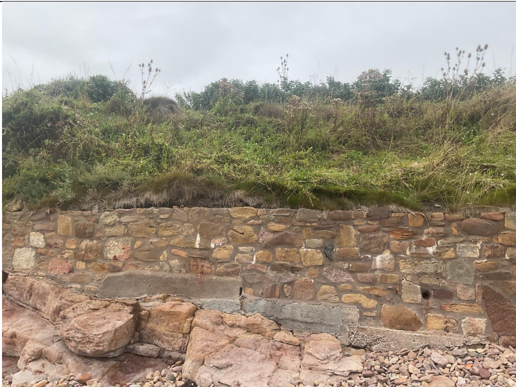
Figure 16- Between ch149-170 a newer section of wall has been Constructed.
