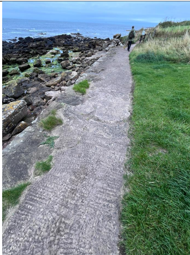
Figure 40- General condition of the path surface between ch236-272.
