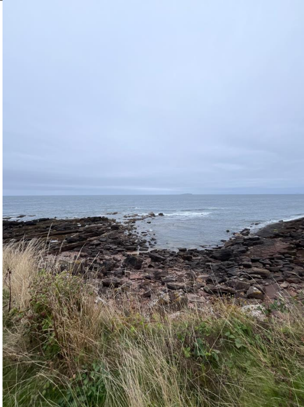
Figure 38- Foreshore area in front of the stretch of wall/coastal path which is largely absent (ch65-ch236).
