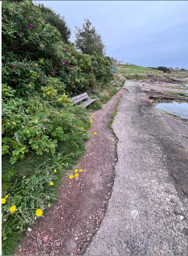
Figure 53- Path surface between ch384-ch414.
