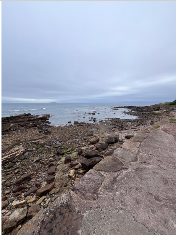
Figure 48-Surface coverage and foreshore materials at ch341-ch349.
