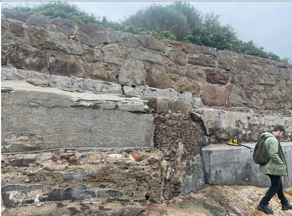
Figure 26- Generalised wall condition for between ch297-ch347. Concrete foundations are much thicker.
