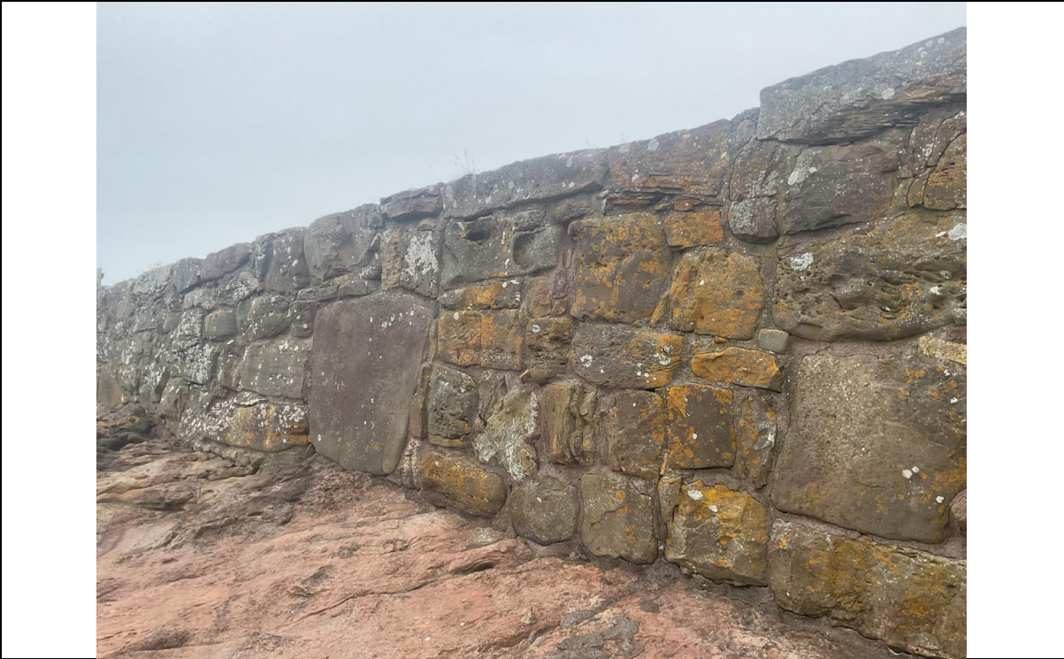
Figure 22- Generally good wall condition between ch239 and ch276.
